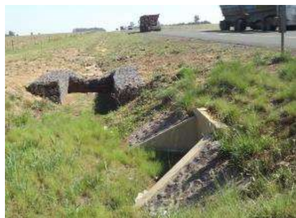
Inlet structures within clear zone
