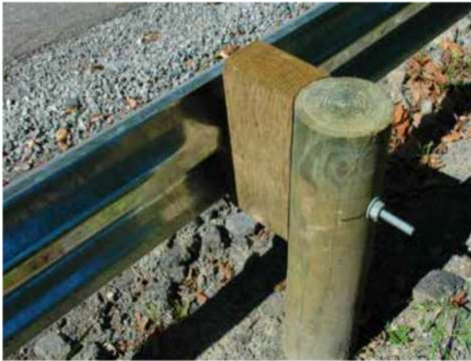
Figure 15: Illustration of Post and Beam Connection
