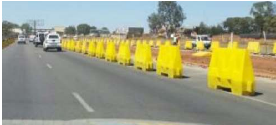
Figure 34: Yellow Plastic Units Used as Delineators
