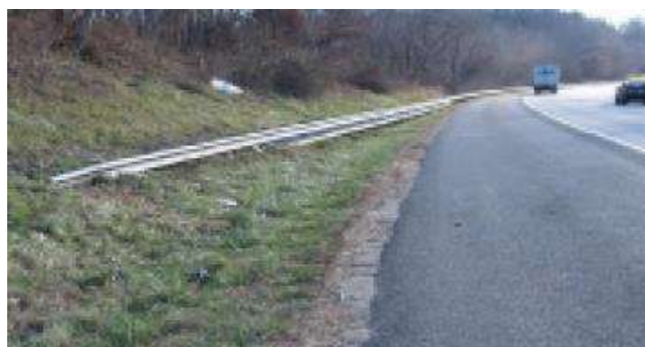
Figure 20: Buried in Backslope Barrier Terminal
