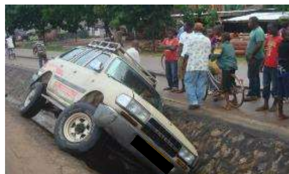
Dangerous deep open drain parallel to road
