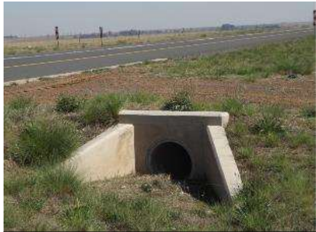
Example of a dangerous drainage structure vs safe structure, at minor road junctions
